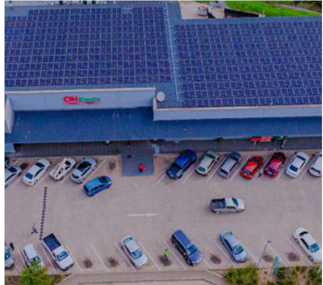
FIGURE 11: Ariel View of 185 kW Rooftop Solar Panels at OK Foods Mbabane
